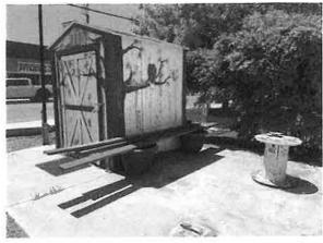
Shed needs to be replaced. Wood is old, Cracked, and splintering.
